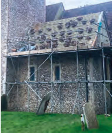
Upper Hardres: south chapel roof being re-tiled & south aisle roof completed
